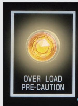
3-phase output from L1, L2 and L3 are monitored. When the current from either of these terminals reaches 80% of the rated output, the warning lamp starts to flash to alert operator to adjust load to a proper level.
