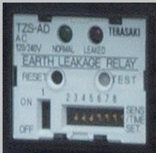
The earth leakage relay detects insulation failure, and automatically cuts the circuit off to prevent electrical shock. The sensitivity current can be adjusted from 30mA to 1000mA with duration of 0.04sec to 2.00sec.
